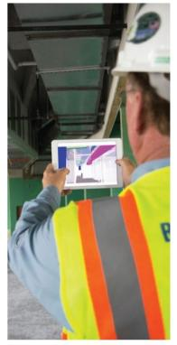
Balfour Beatty is looking to LiDAR laser scanner-enabled tablets to help facilitate more digitally connected jobsites.
