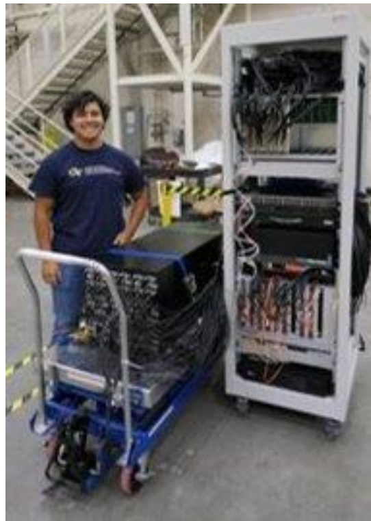
Figure 1. ROADSTR refurbished and collecting data
