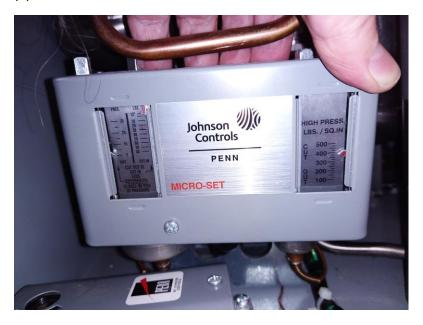
Switch in its original setting. The middle switch shows a shutoff pressure of 12"Hg. This should be set to 0 or slightly positive using the set-screw.
