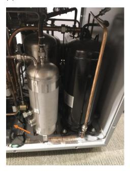
The switch is in the lower left hand corner. Its front side is facing the wall so that the dials are not visible. The switch needs to be unbolted from the floor.
